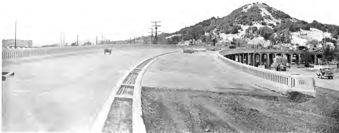
View of highway viaduct through San Rafael, which is nearing completion
